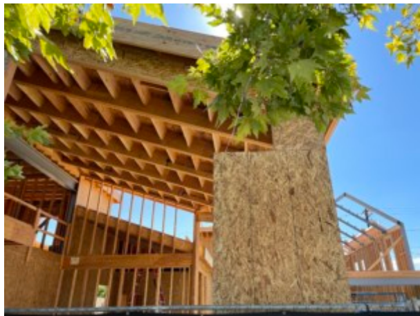
Shasta Bike Depot under construction
